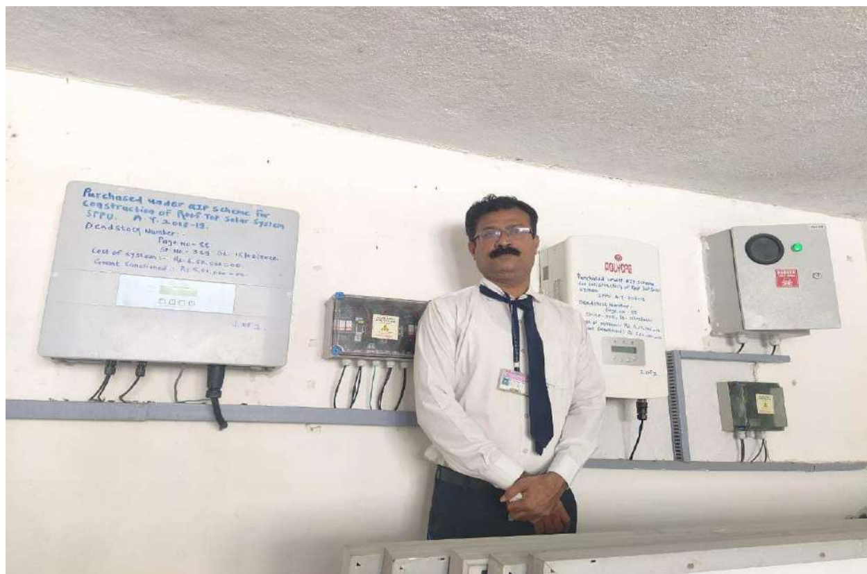
Photo 3- Solar Panel Details Installed with Project Coordinator Dr.Y. S. Angal (HOD (E&TC))
