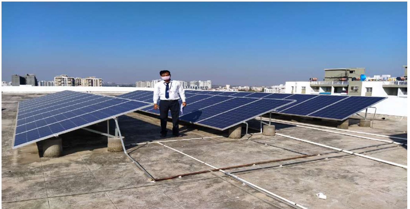
Photo 2: Solar Panel Installed with Project Coordinator-Dr.Yogesh S. Angal(HOD(E&TC))
